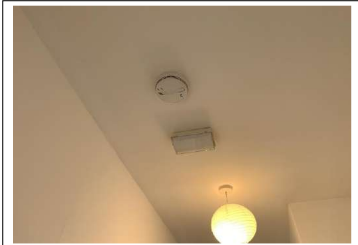
Location – Hallway Ceiling
