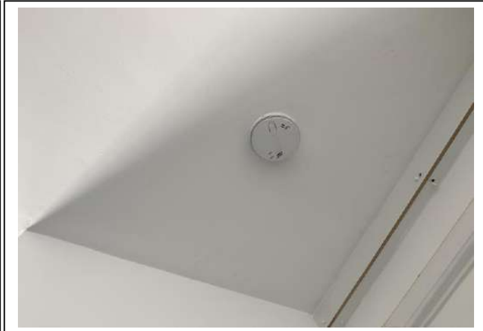
Location – Lounge Ceiling
