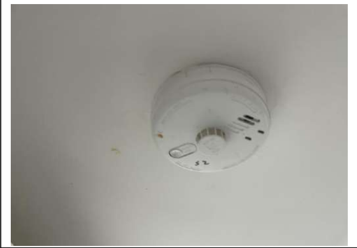
Location – Kitchen Ceiling
