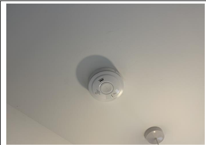
Location – Hallway Ceiling
