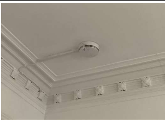
Location – Lounge Ceiling
