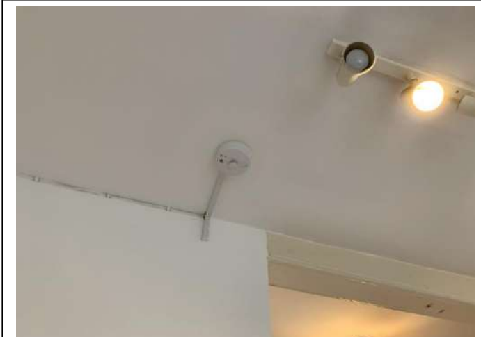
Location – Kitchen Ceiling
