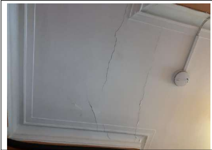
Location – Hallway Ceiling
