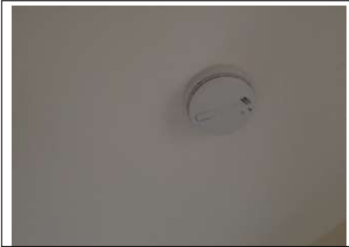
Location – Hallway Ceiling
