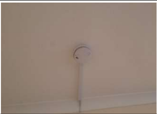
Location – Lounge Ceiling
