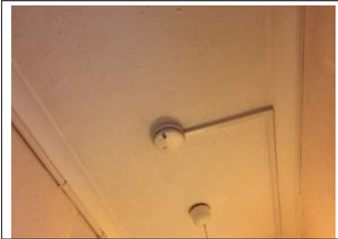
Location – Hallway Ceiling
